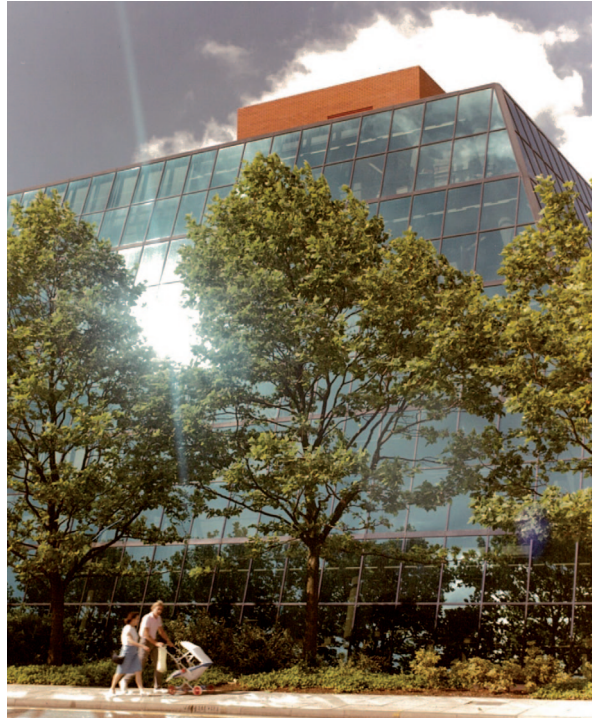
Figure 39: Solar dazzle reflected from a glazed façade
