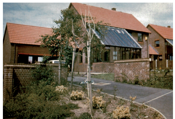
Figure 32: At Willow Park, Chorley, careful road layout design means that all the passive solar homes can have a southerly orientation
