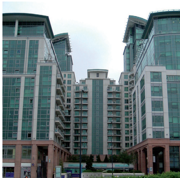
Figure 7: A tunnel effect can occur if a window has projecting wings on both sides of it. In this development in South London (architects Broadway Malyan), the windows have been increased in size to compensate.
