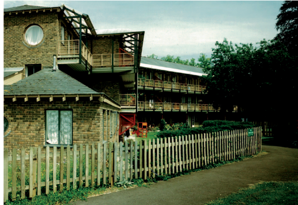
Figure 24: In this housing association scheme, solar shading is provided by balconies and overhangs
