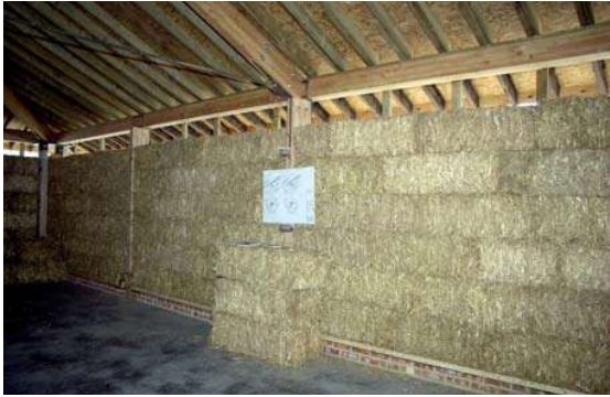
Figure 6: Six courses of straw bales laid in stretcher bond with the seventh about to be added (Courtesy of Mike Beckett/Collins & Beckett)
