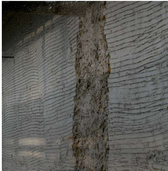
Figure 10: Second coat of render has been applied (Courtesy of Mike Beckett/Collins & Beckett)
