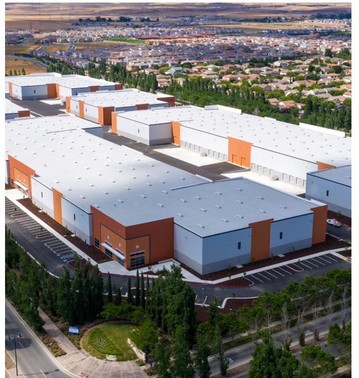
Mountain Technology Center, California
